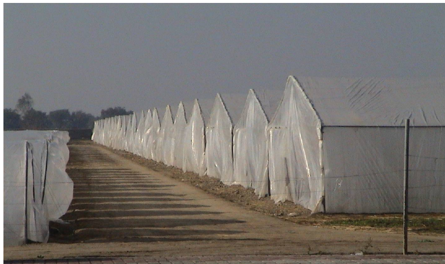
Figure 3-4: Picture of High Tunnel 6
