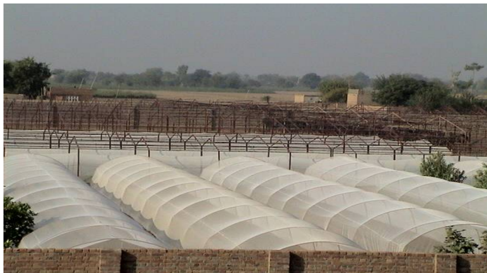
Figure 3-5: Support structure in High tunnels
